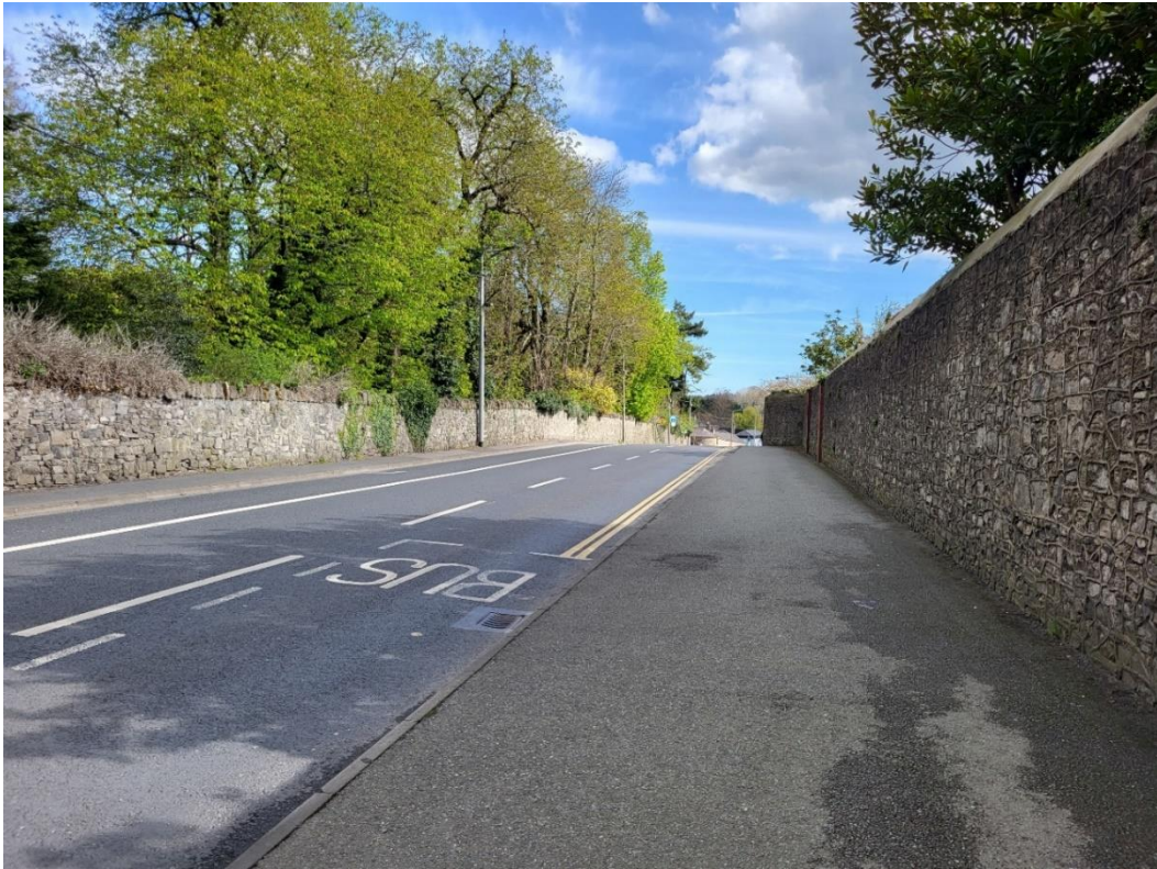
Figure 1 Looking towards Lucan village, the hump in the Leixlip Road as it passes over the tunnel is evident. Lucan Demesne is located on the left, while its walled garden, now the Orchard Estate, is on the right. The bow-fronted projection that houses the stairs to the tunnel from the orchard is visible on the background. This was once mirrored on the far side of the road.
