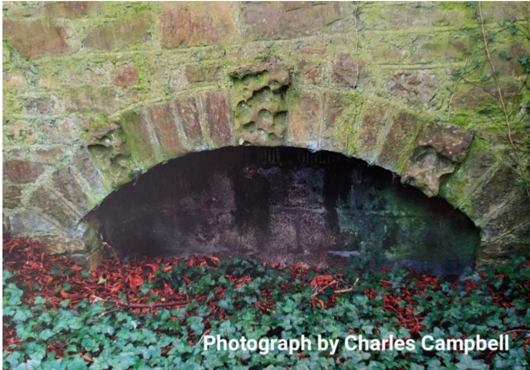
Figure 12 A photograph of the Demesne archway in Desmond Guinness' book on Lucan House shows the top section of the blocked-up archway free of overgrowth. The keystone and two of the Voussoirs are cut from naturally rusticated limestone, a feature which is found throughout the grounds of the Demesne and dating to the 18 th century. Source: Lucan House by Desmond Guinness.
