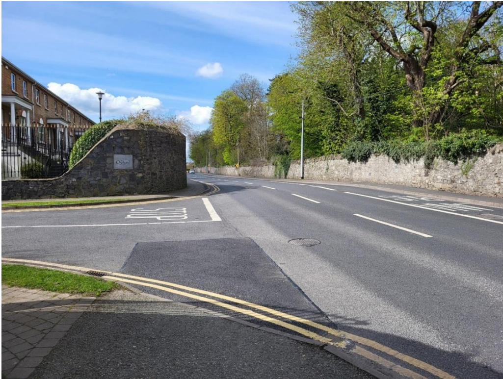
Figure 7 View of the hump over the tunnel looking away from Lucan Village. The bow-fronted projection in the Orchard wall has been incorporated into the entrance of the walled estate, with a new section of wall with railings following the curve of the original projection. This entrance is new, with the original entrance (hidden from view behind the projection) being blocked up.
