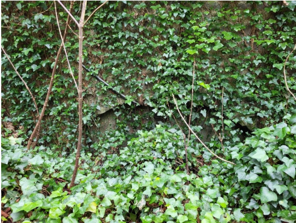
Figure 10 The archway set within the boundary wall of the Demesne was almost completely obscured, being half buried and covered by overgrowth. Originally set within a bow-fronted projection similar the one on the orchard side, the arch was relocated to its current location when the wall of the Demesne was straightened. This archway was blocked up in the 1930's when the lands of the walled garden where sold, breaking the link which had joined the two for centuries. The use of the tunnel to house telecommunications is highlighted by the thick cable exiting through the top of the tunnel.
