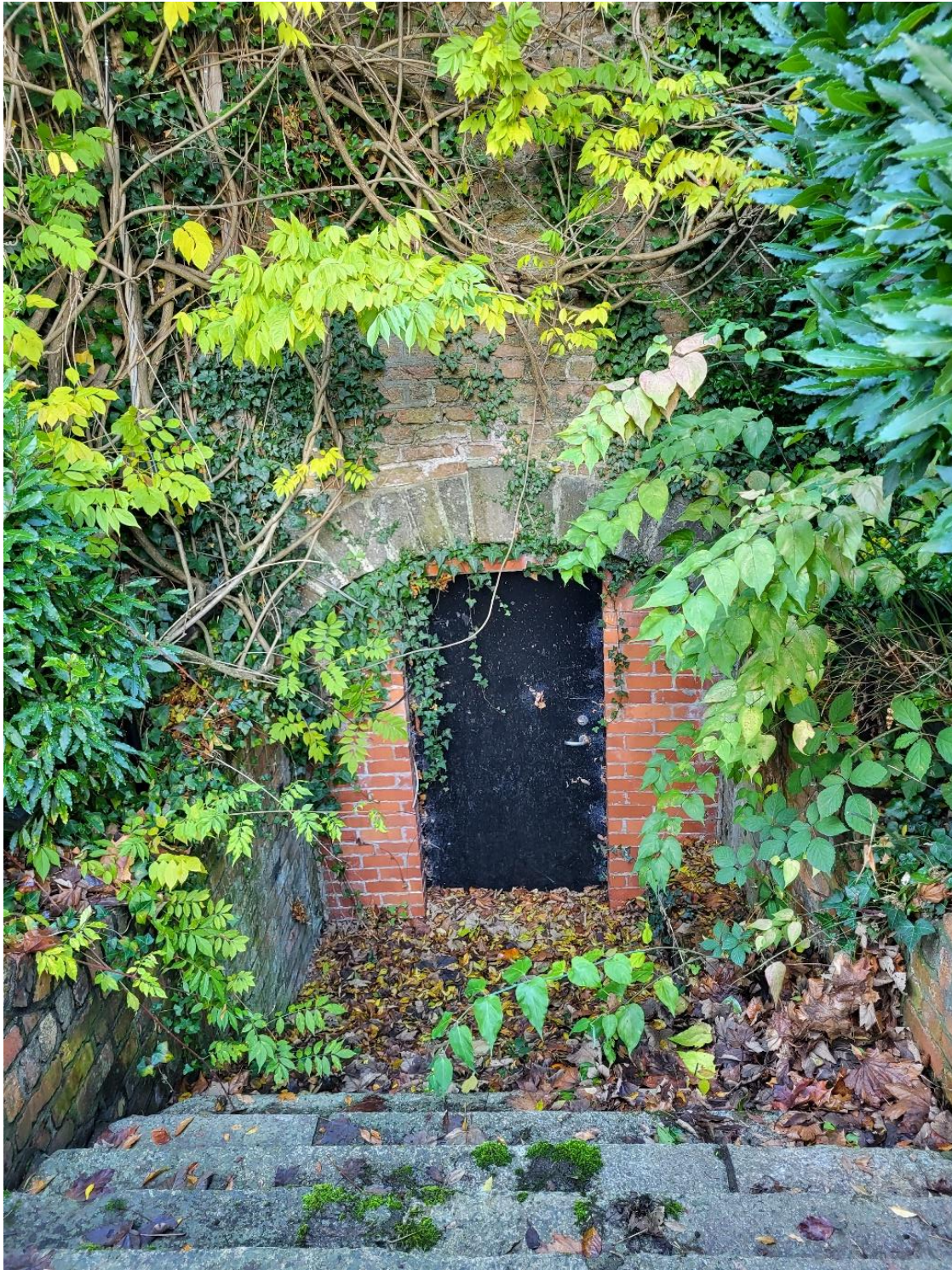
Figure 9 The original archway to the tunnel, located within the projection of the Orchard wall. Originally a wide, open archway, it was later bricked up with a doorway being inserted to prevent access. The flight of stone steps that lead down to the archway have been preserved. The arch is formed by plain cut stone voussoirs.
