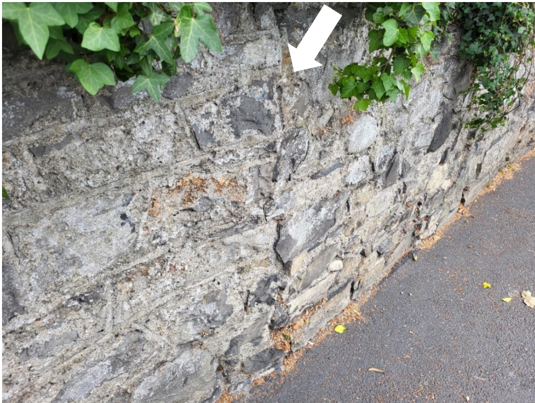
Figure 6 The random rubble masonry of the original boundary on the right, with the neater blockwork of the infilled section on the left. The seam between the two runs in a straight line down the middle of the wall.
