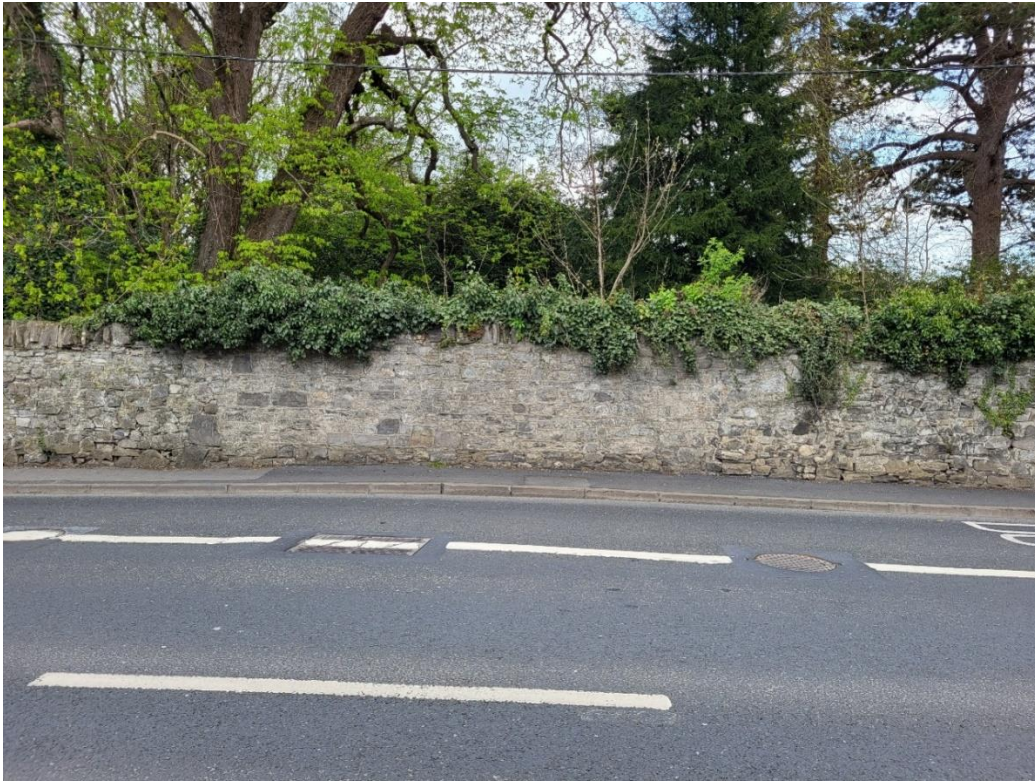
Figure 3 The boundary wall of the Demesne once had a bow-fronted projection like the one in the Orchard wall, however it was removed, and the boundary wall straightened. Telecommunication services now occupy a section of the tunnel, the access points to which can be seen at the crown of the hump in the middle of the of the road. A manhole to the right shows that the modern sewer system also runs down the middle of the road, cutting through the tunnel.
